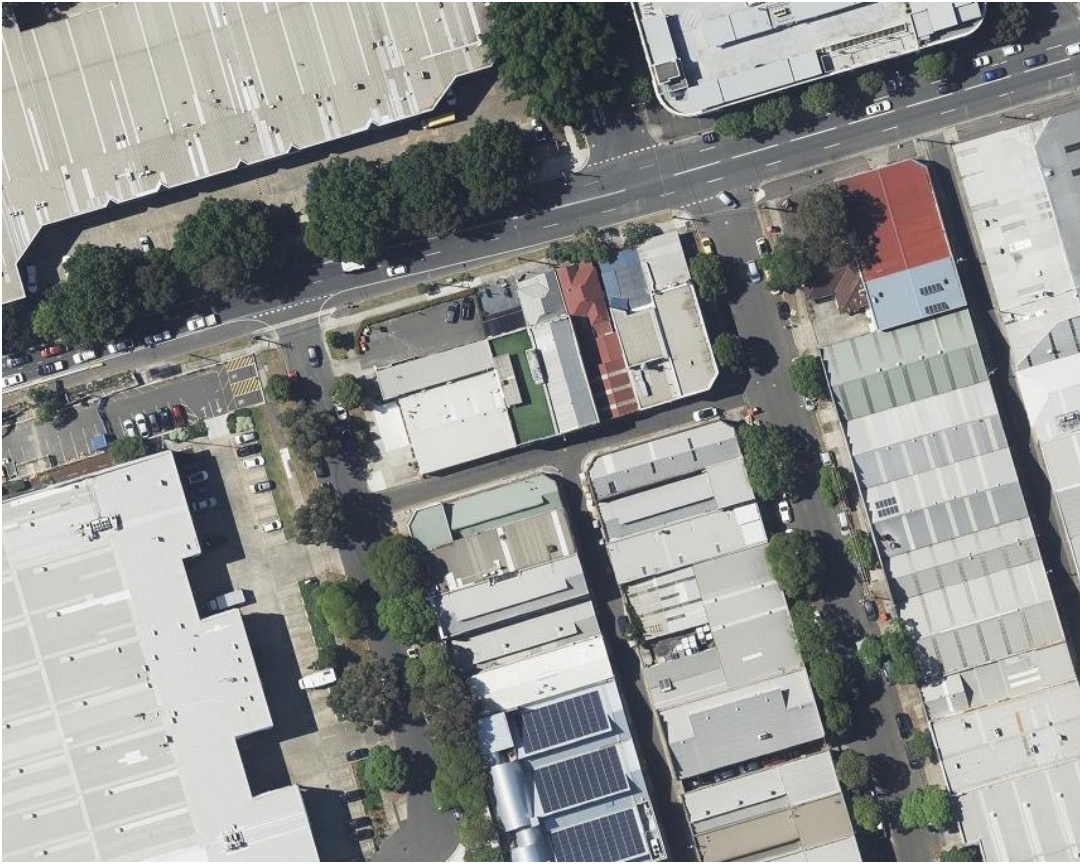
2024 aerial image of subject site.
